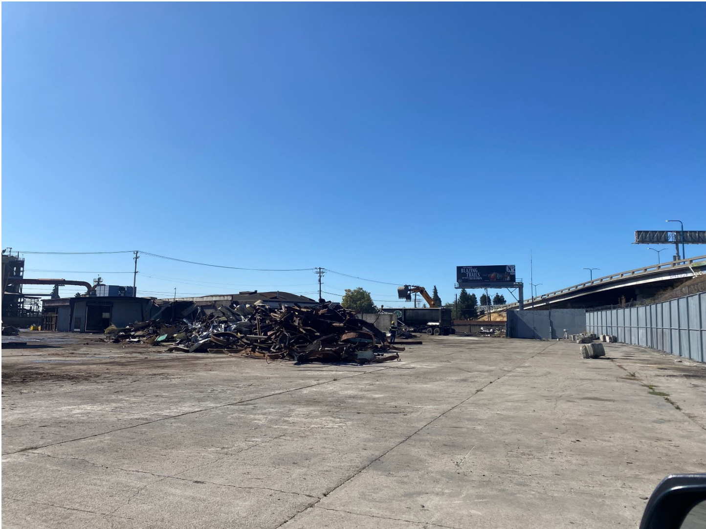
Photo 1: Facing south, loading trucks with debris from the sand storage area.
