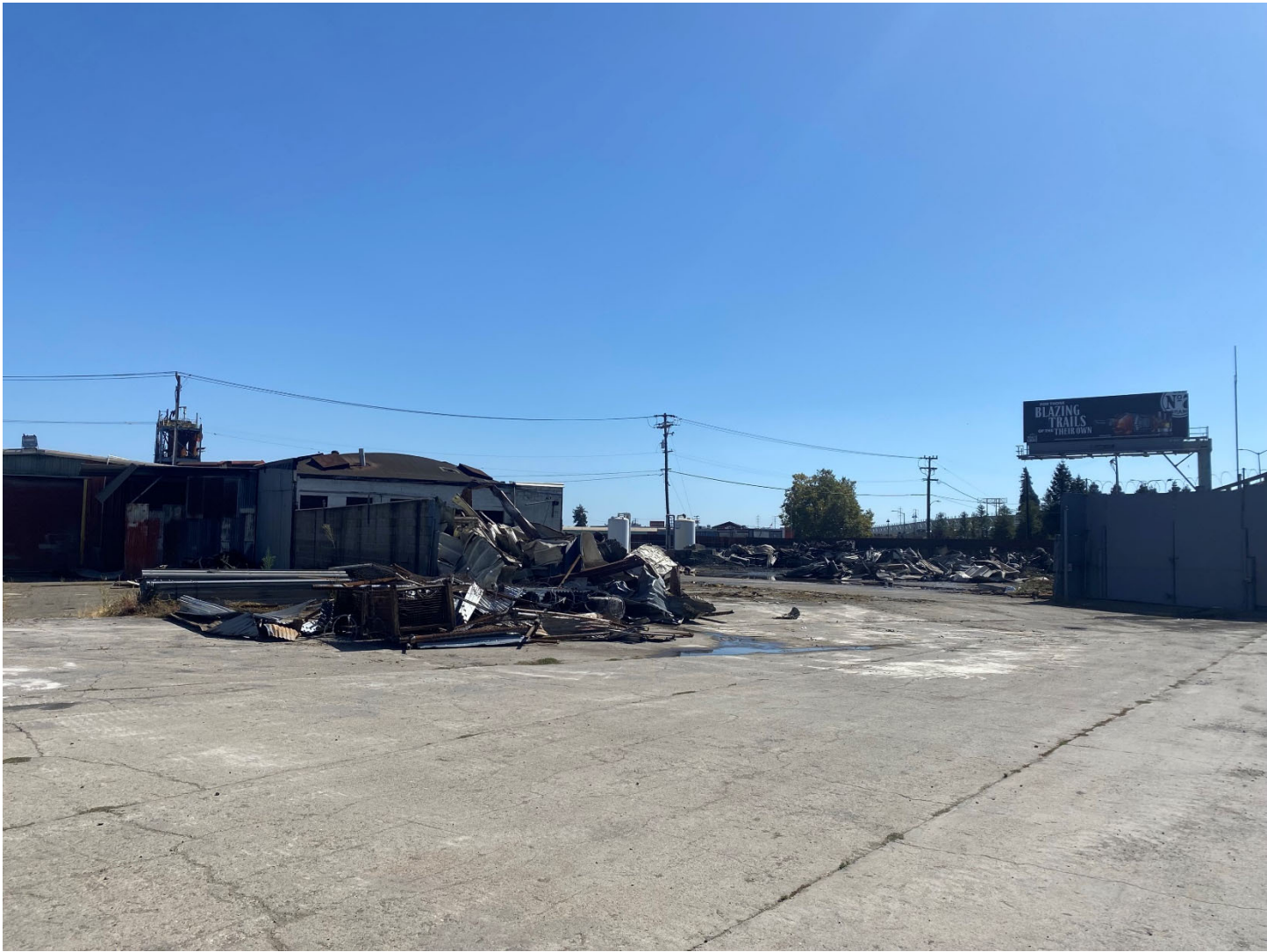
Photo 3: Demolition of the Special Finishing building (left) and Sand Storage Area (right).
