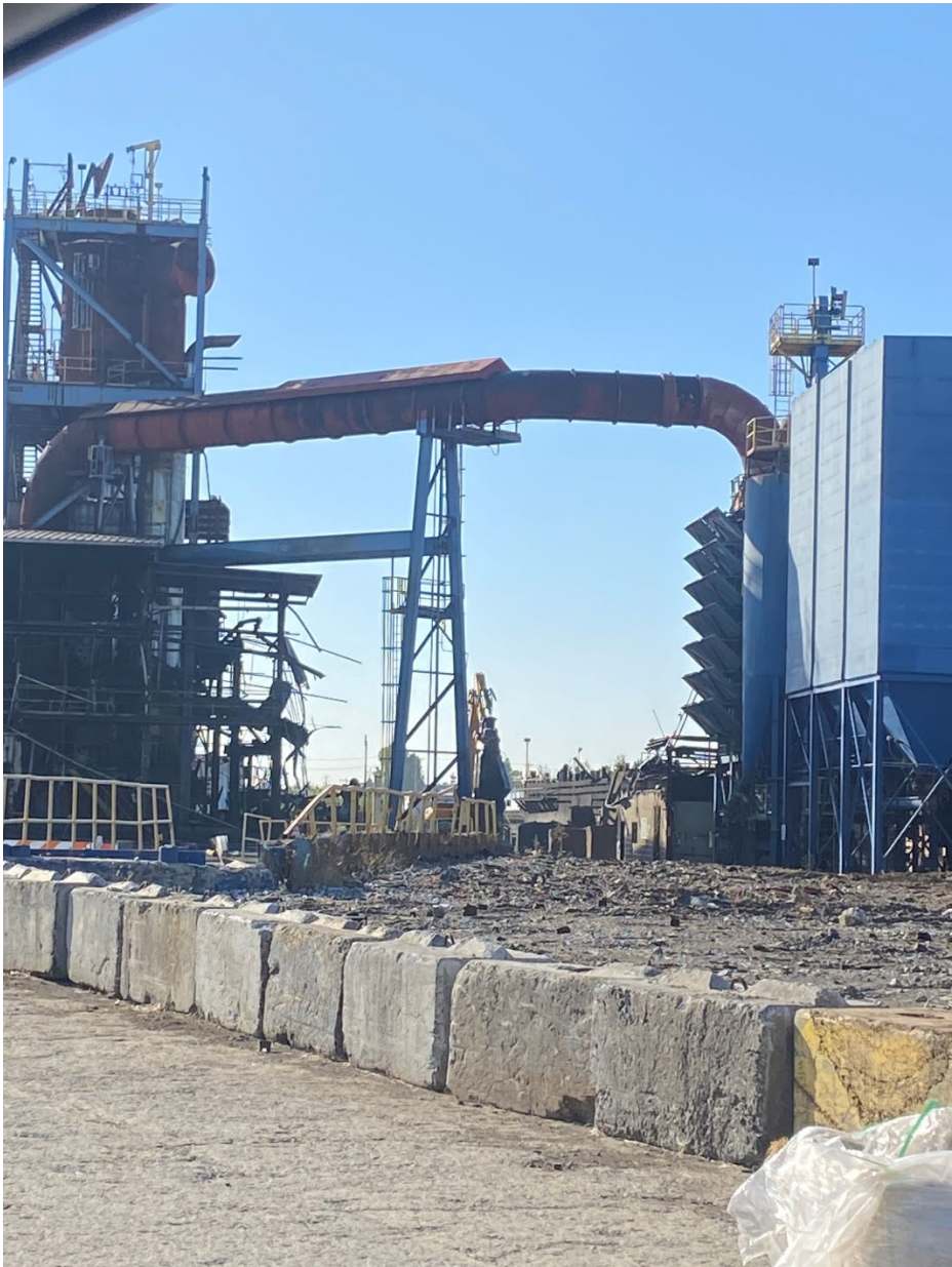
Photo 2: Facing southeast. Demolition of the catwalk on the southwest portion of the main building.
