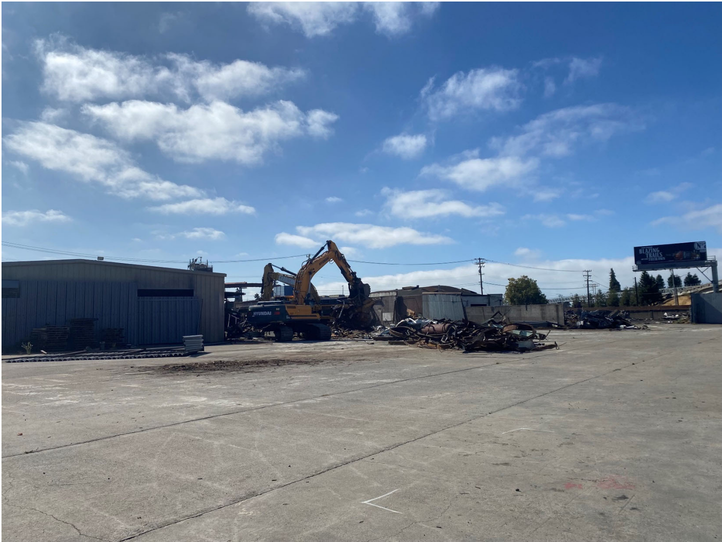
Photo 2: Looking south. Demolition work in the vicinity of the former Special Finishings area (northwestern portion of Site).
