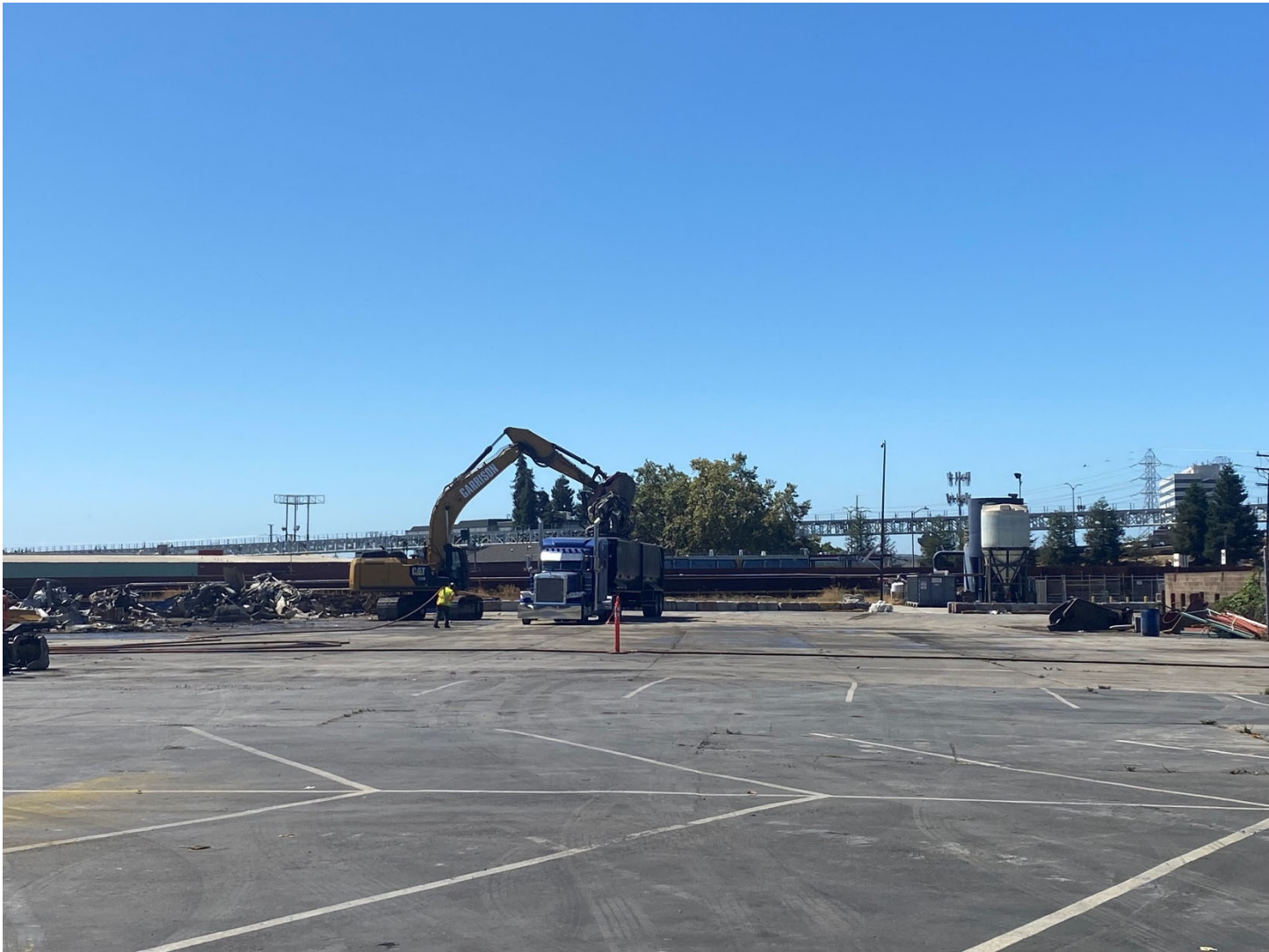
Photo 2: Loading trucks with demolition debris from the rolling stock shop, maintenance and stockroom buildings.
