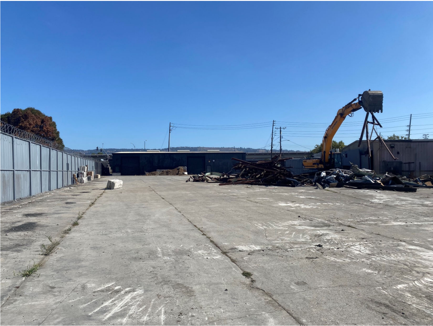
Photo 3: Looking northeast towards San Leandro Street. Forming stockpiles in northwestern portion of Site.
