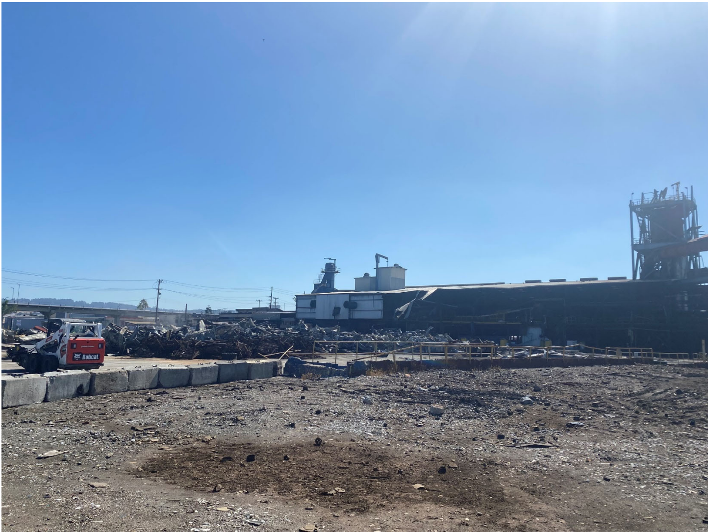
Photo 1: Completed demolition of the Maintenance and Stockroom buildings.
