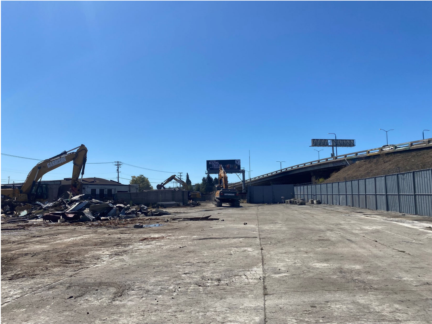
Photo 3: Facing south, demolition progress in the vicinity of the special finishings area.
