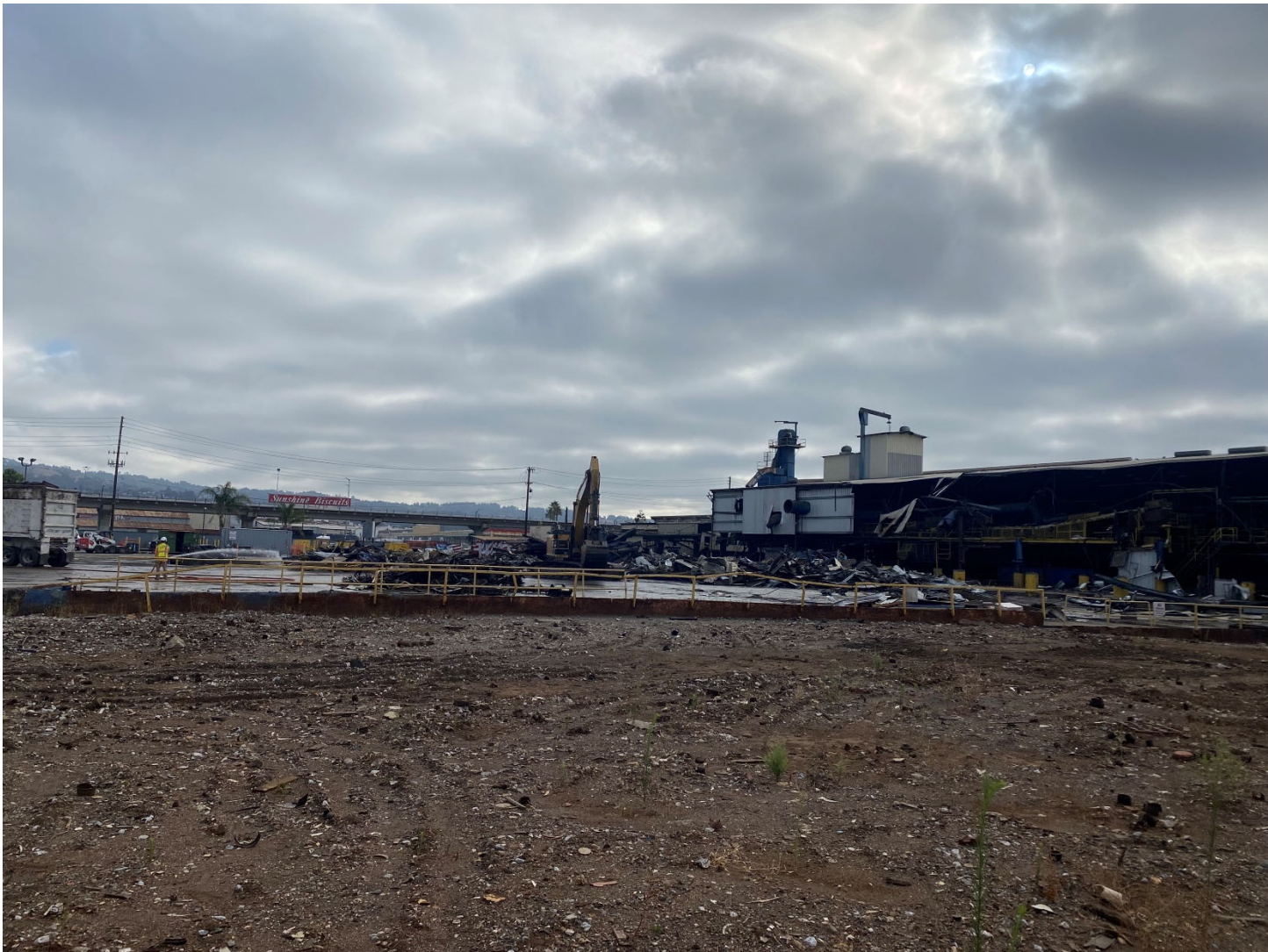
Photo 1: Looking east. Debris stockpiles from former stockroom and maintenance area (central portion of Site).
