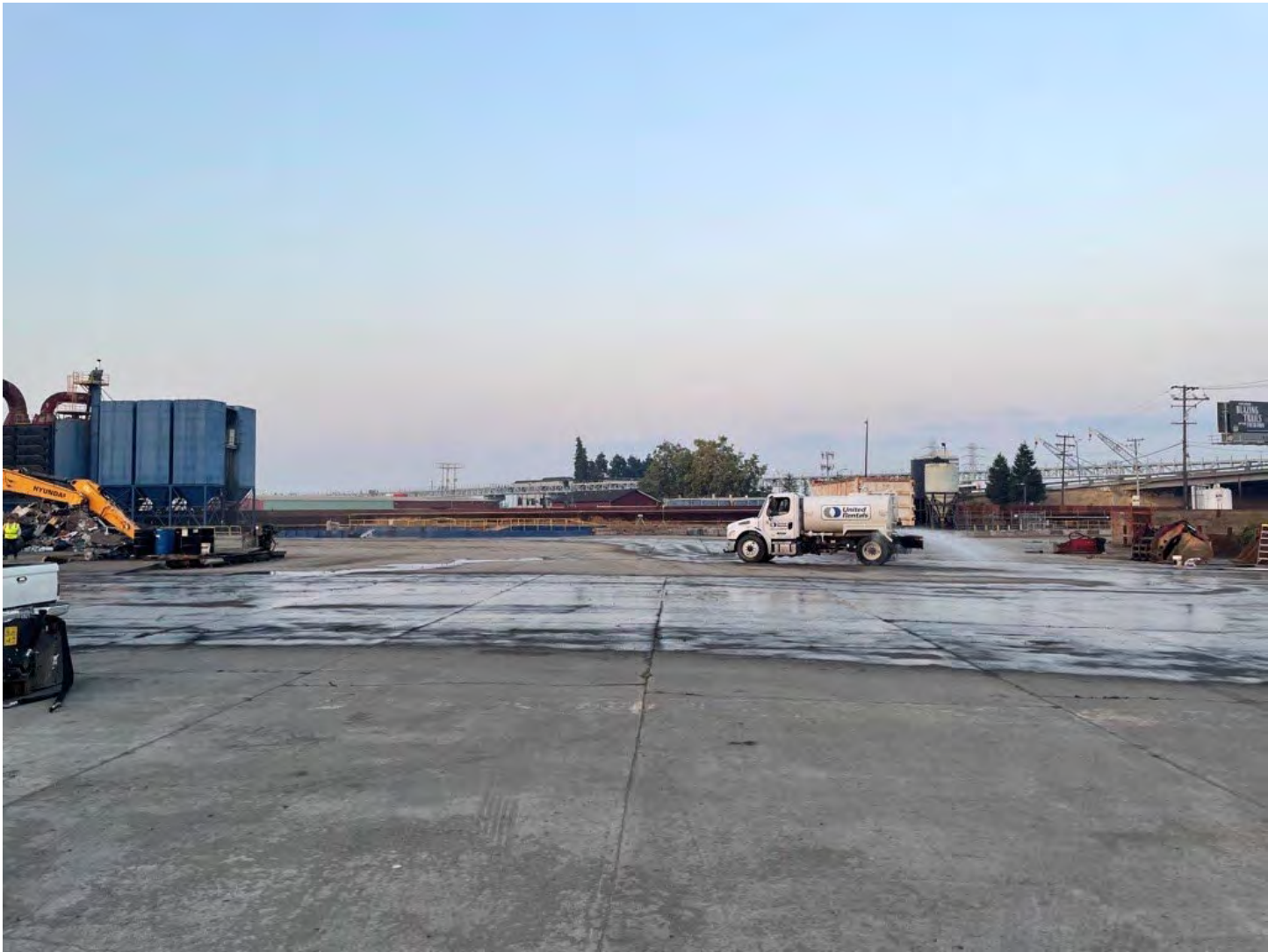
Photo 1: Facing west southwest, dust suppression on truck path.
