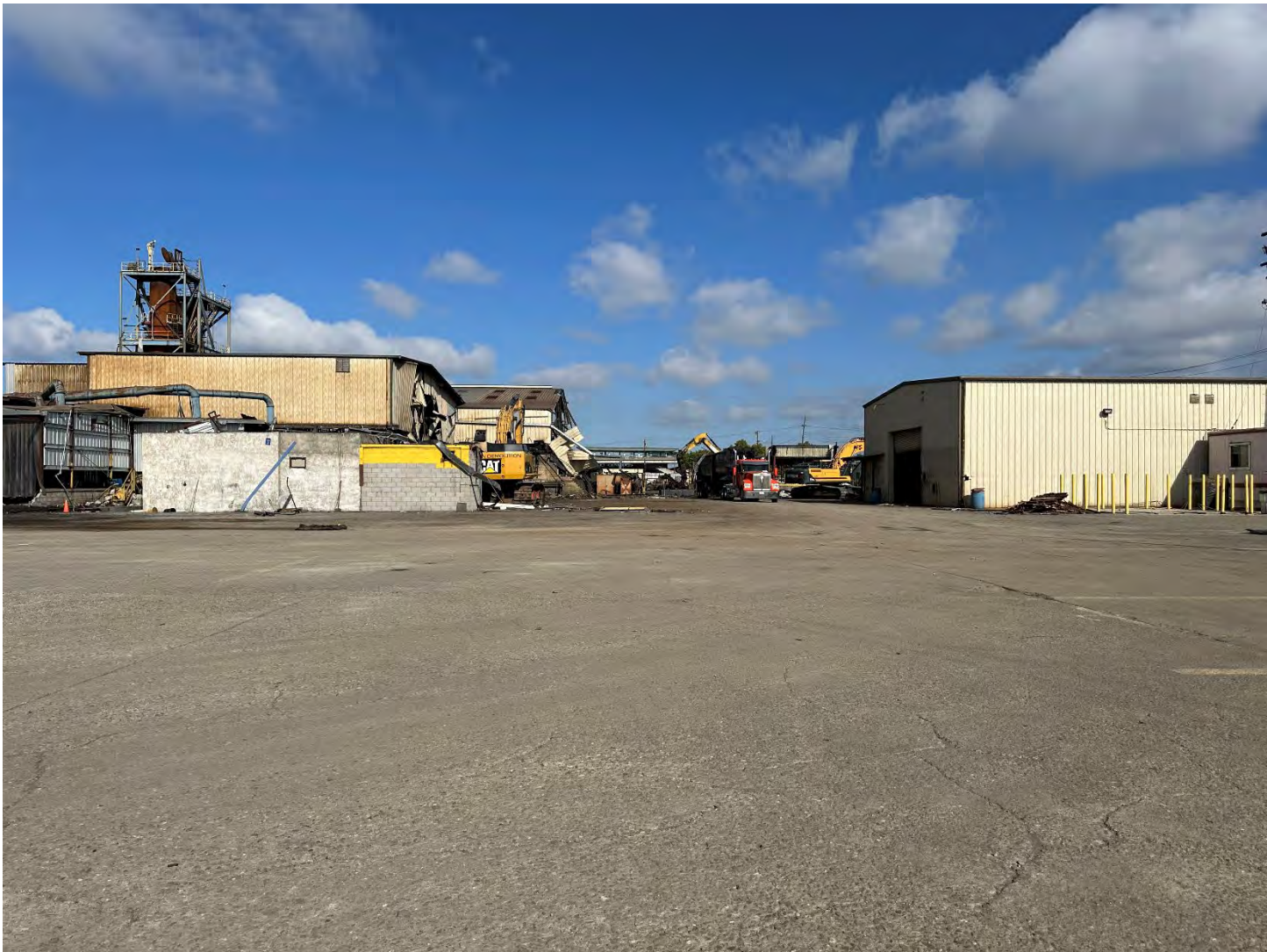
Photo 2: Facing northwest, loading trucks with demolition debris from central portion of main building.
