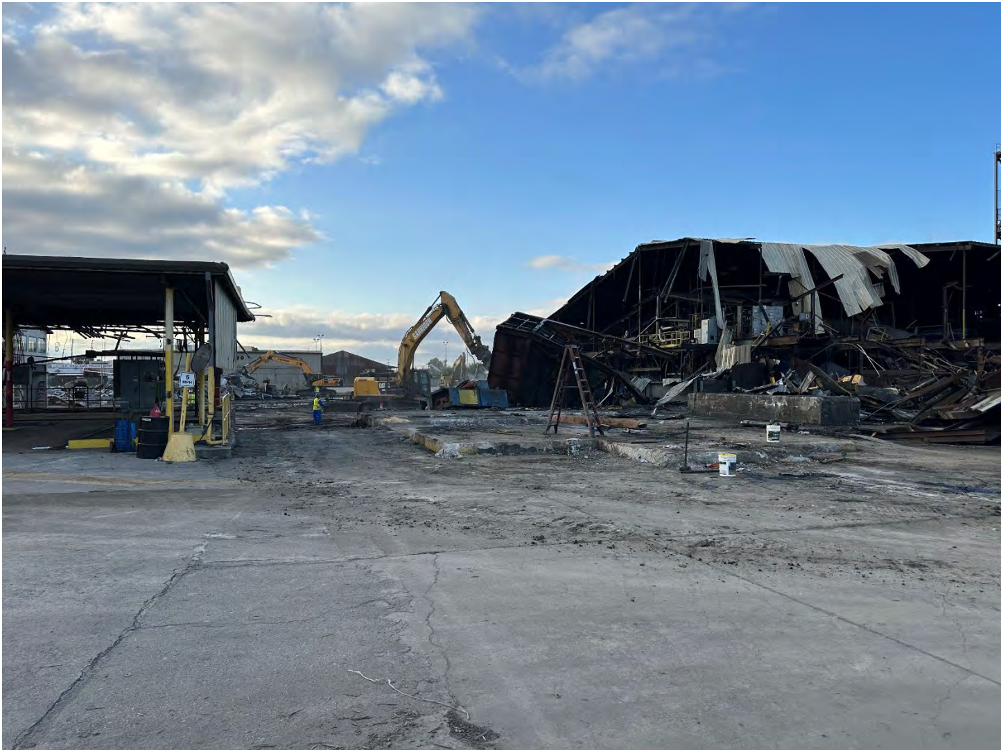
Photo 1: Facing southeast, demolition of the central portion of the former main building.
