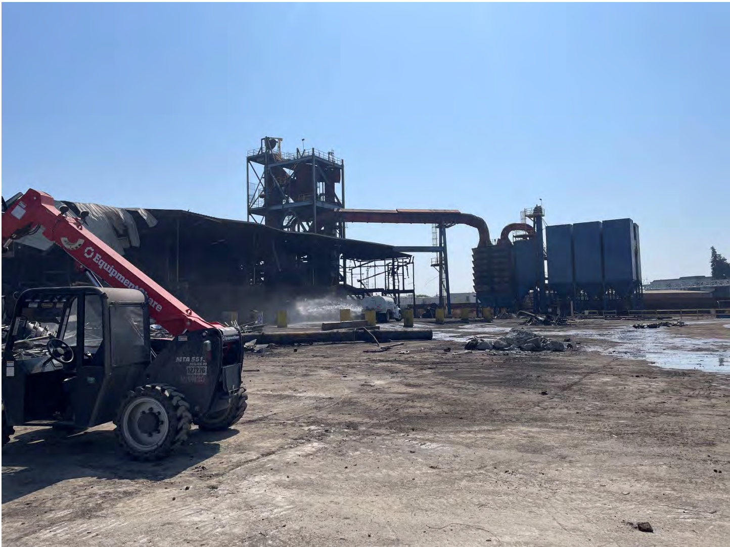
Photo 2: Facing southwest, dust suppression on truck path.
