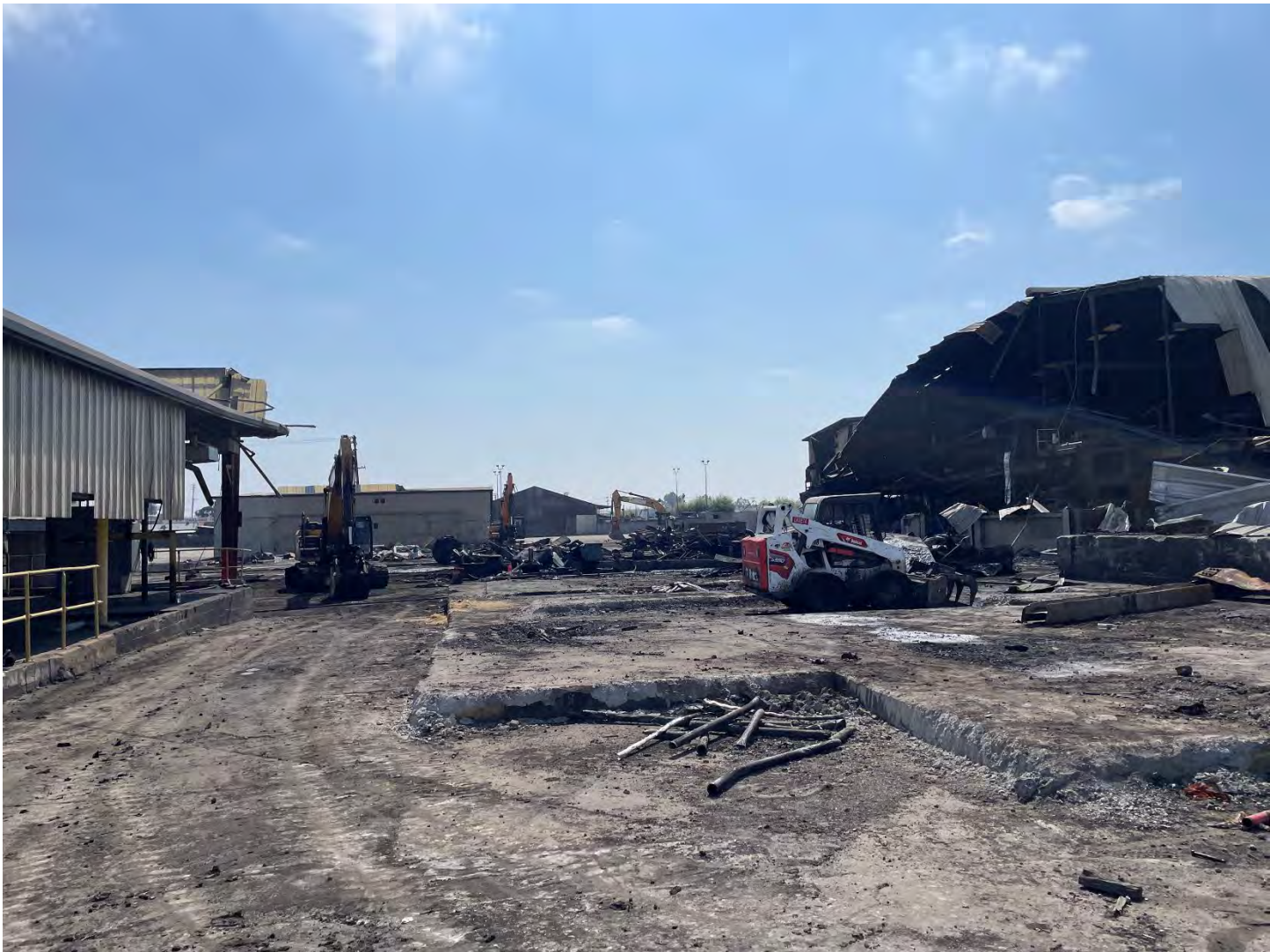
Photo 3: Facing southeast, demolition progress of the former main facility.
