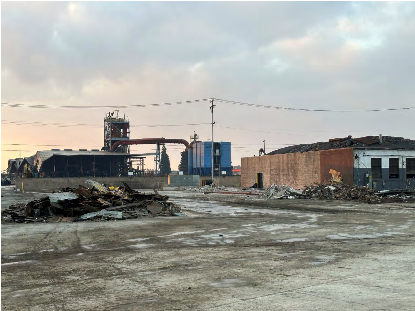
Photo 2: Facing south, continued demo preparation of special finishing facility.
