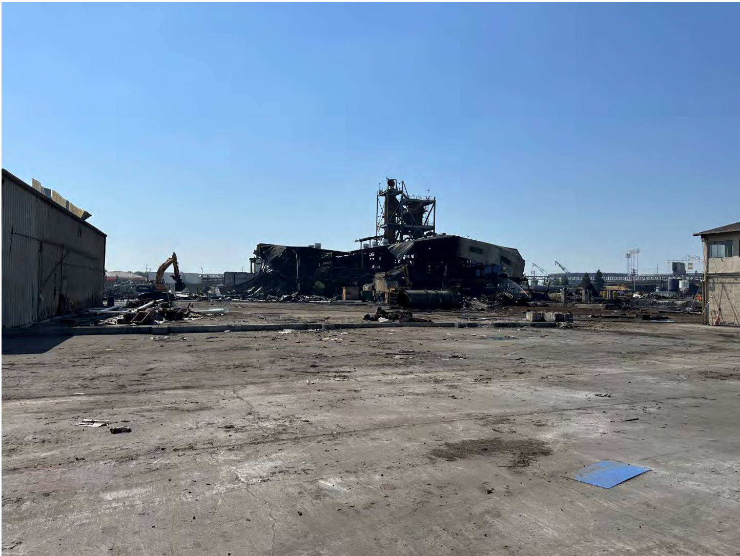
Photo 3: Facing southwest, demolition progress on east side of main building.
