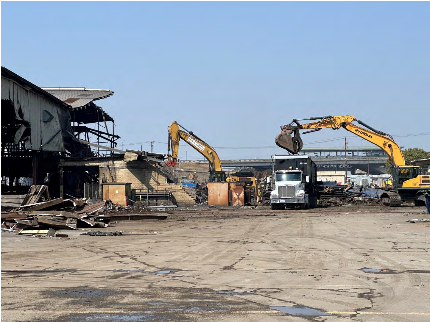
Photo 3: Facing northwest, demolition progress of the former main facility and off hauling debris.
