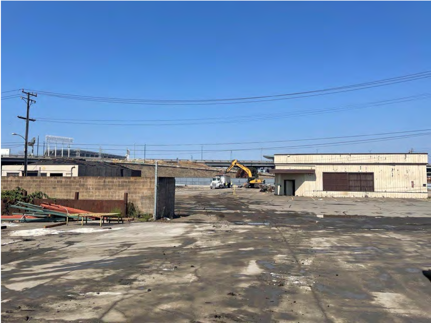
Photo 4: Facing southwest, loading trucks with demolition debris from former casing storage.
