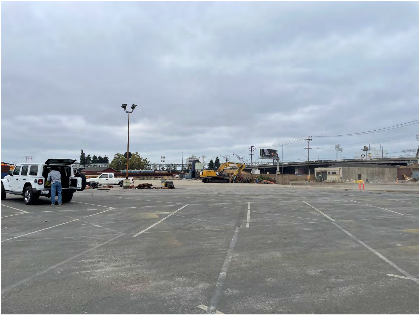
Photo 4: Facing west northwest, hot work activities on the southeast side of the former casing storage building.
