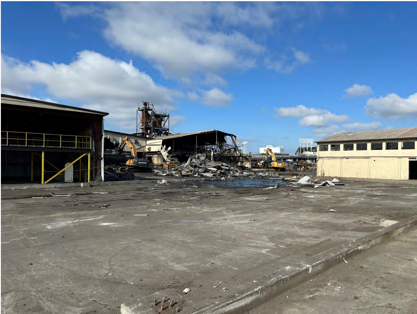
Photo 3: Facing west, demolition progress on east side of main building.
