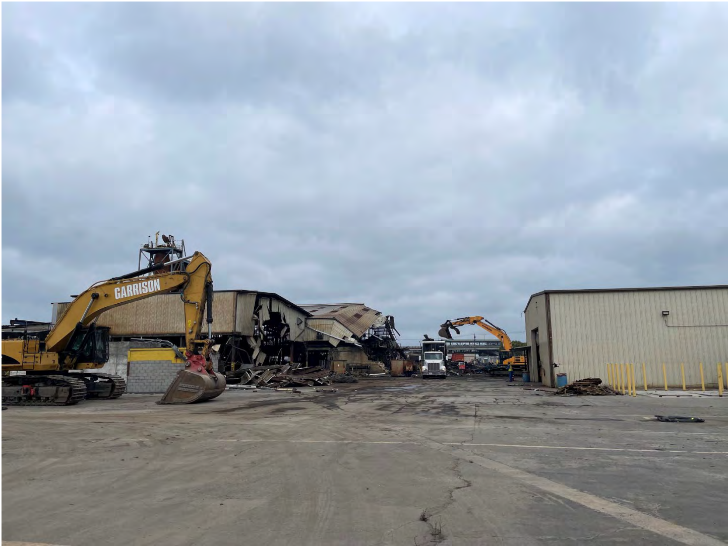
Photo 1: Facing northwest, loading trucks with demolition debris from the former main facility.
