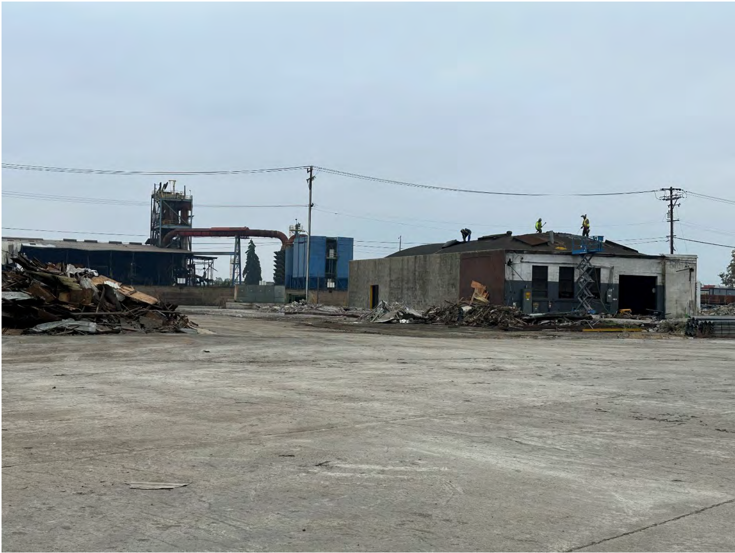
Photo 2: Facing south, demolition prep. on the roof of the remaining Special Finishing building.
