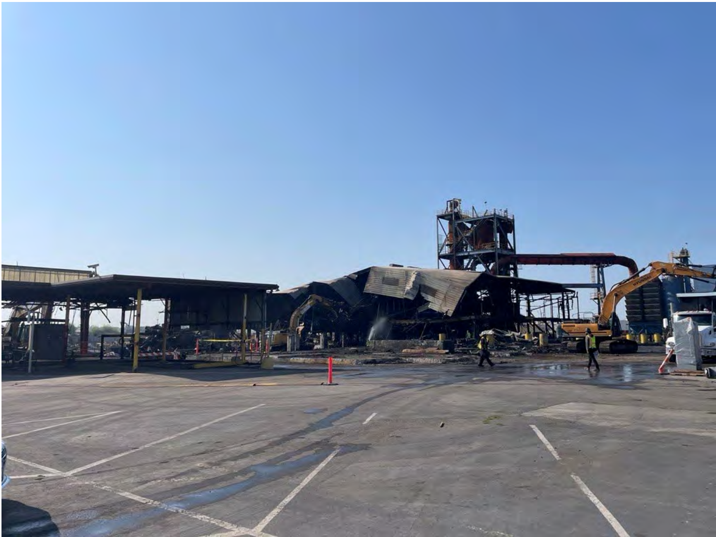
Photo 2: Facing south, demolition progress in the vicinity of the former main facility.
