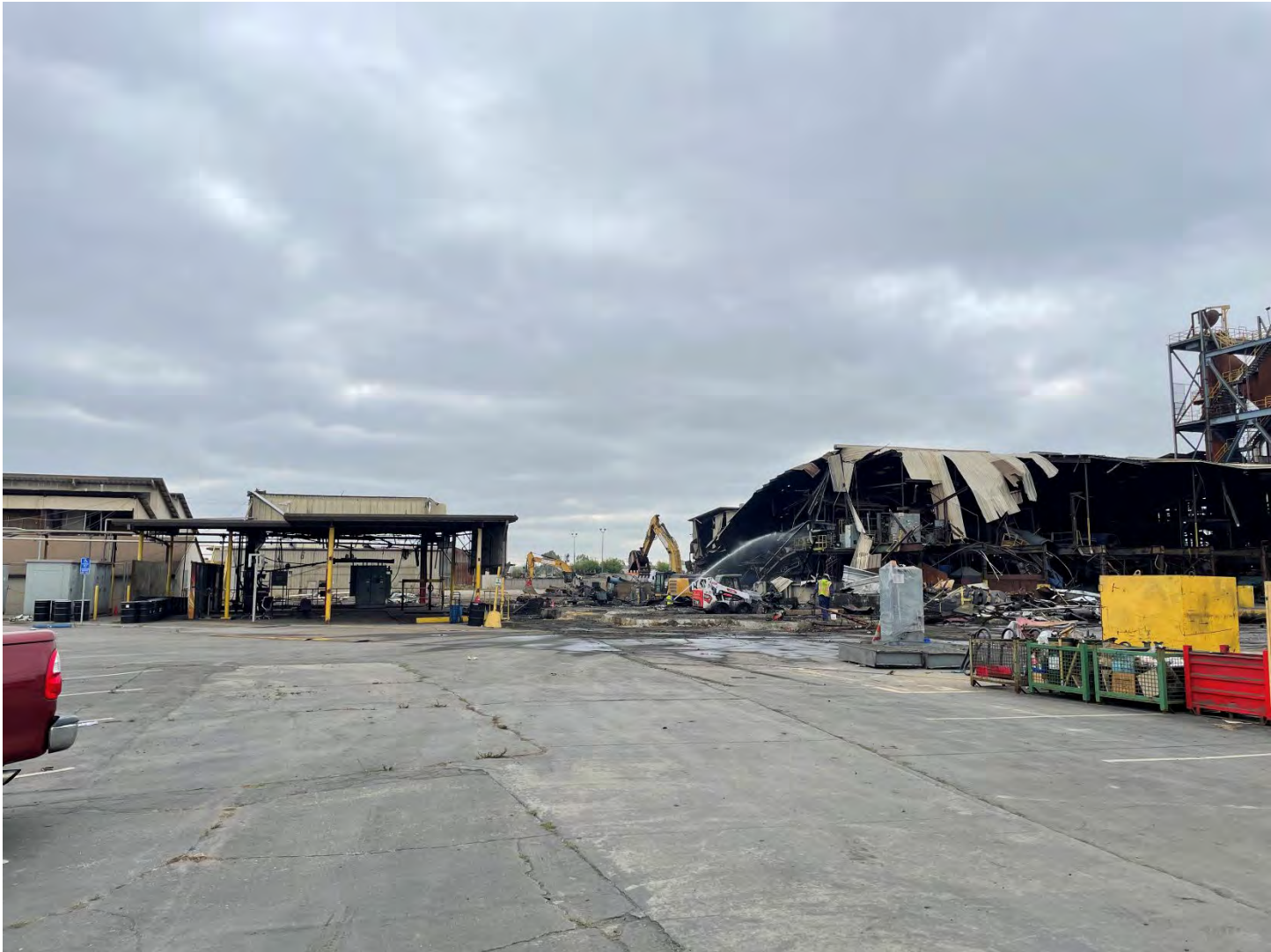
Photo 5: Facing west southeast, demolition of former main facility.
