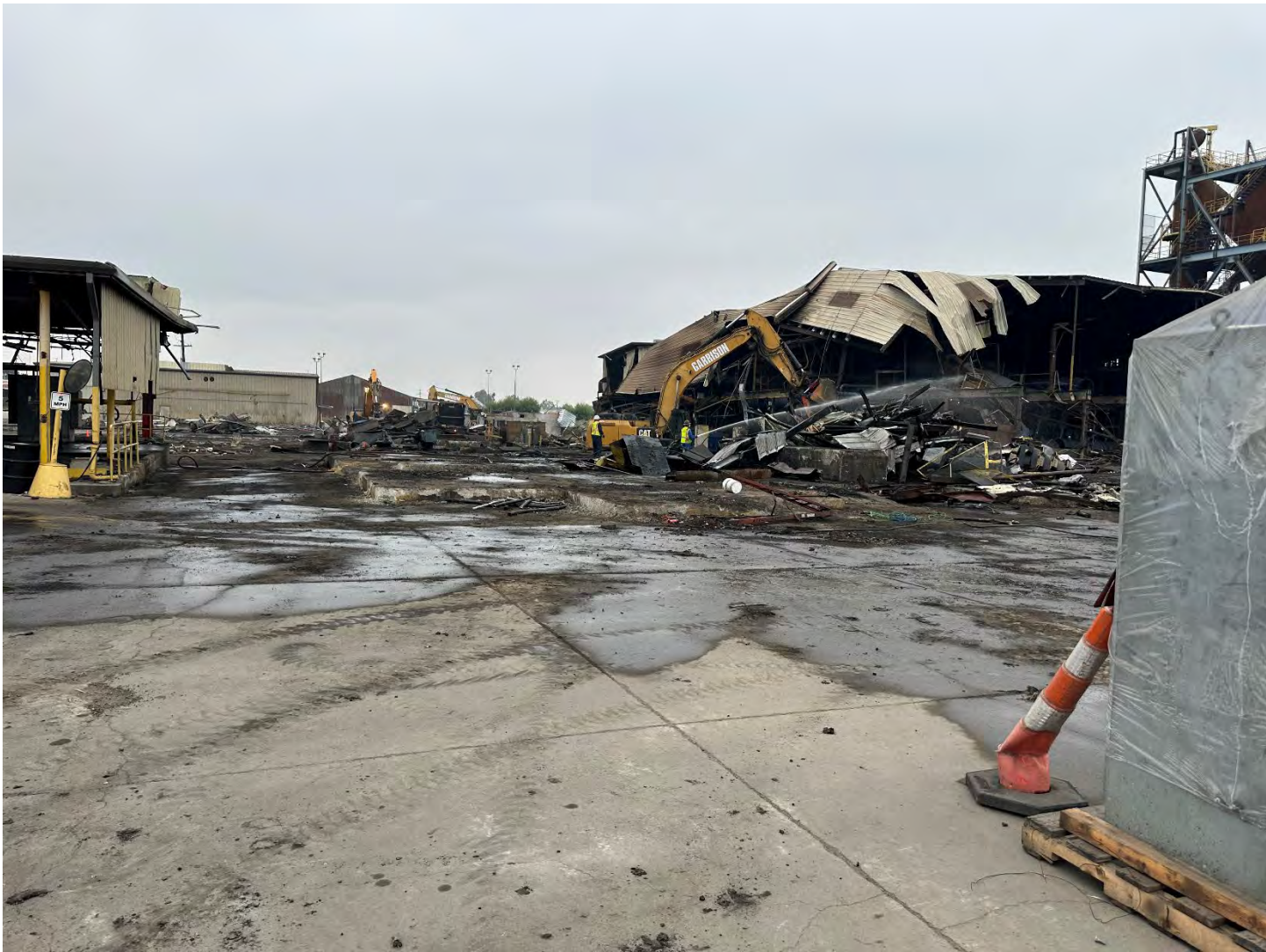
Photo 1: Facing south, continued demolition and dust mitigation of southeast portion of former Main Facility.
