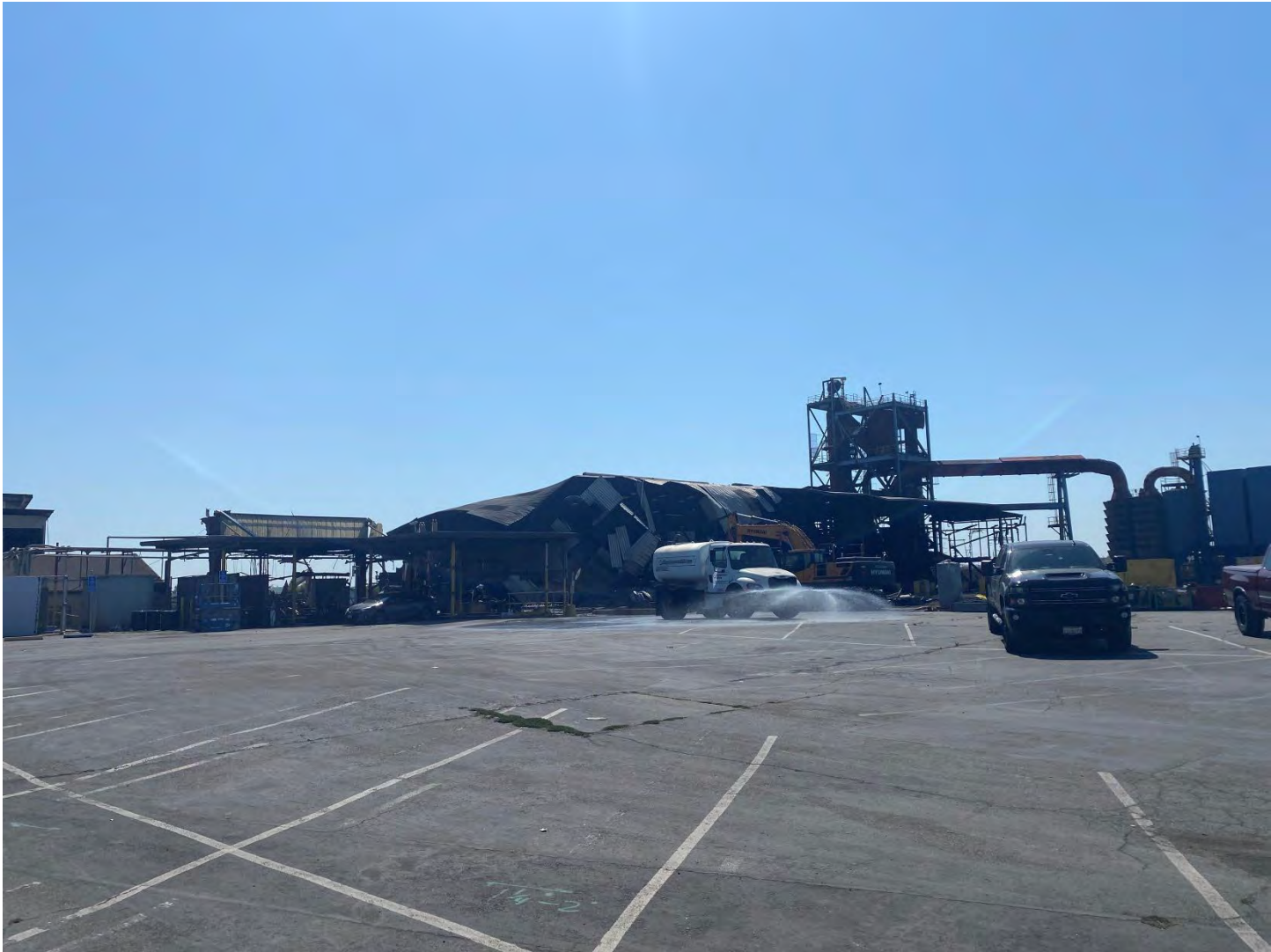
Photo 4: Facing south, dust suppression with water truck following collapse of structure on main facility.
