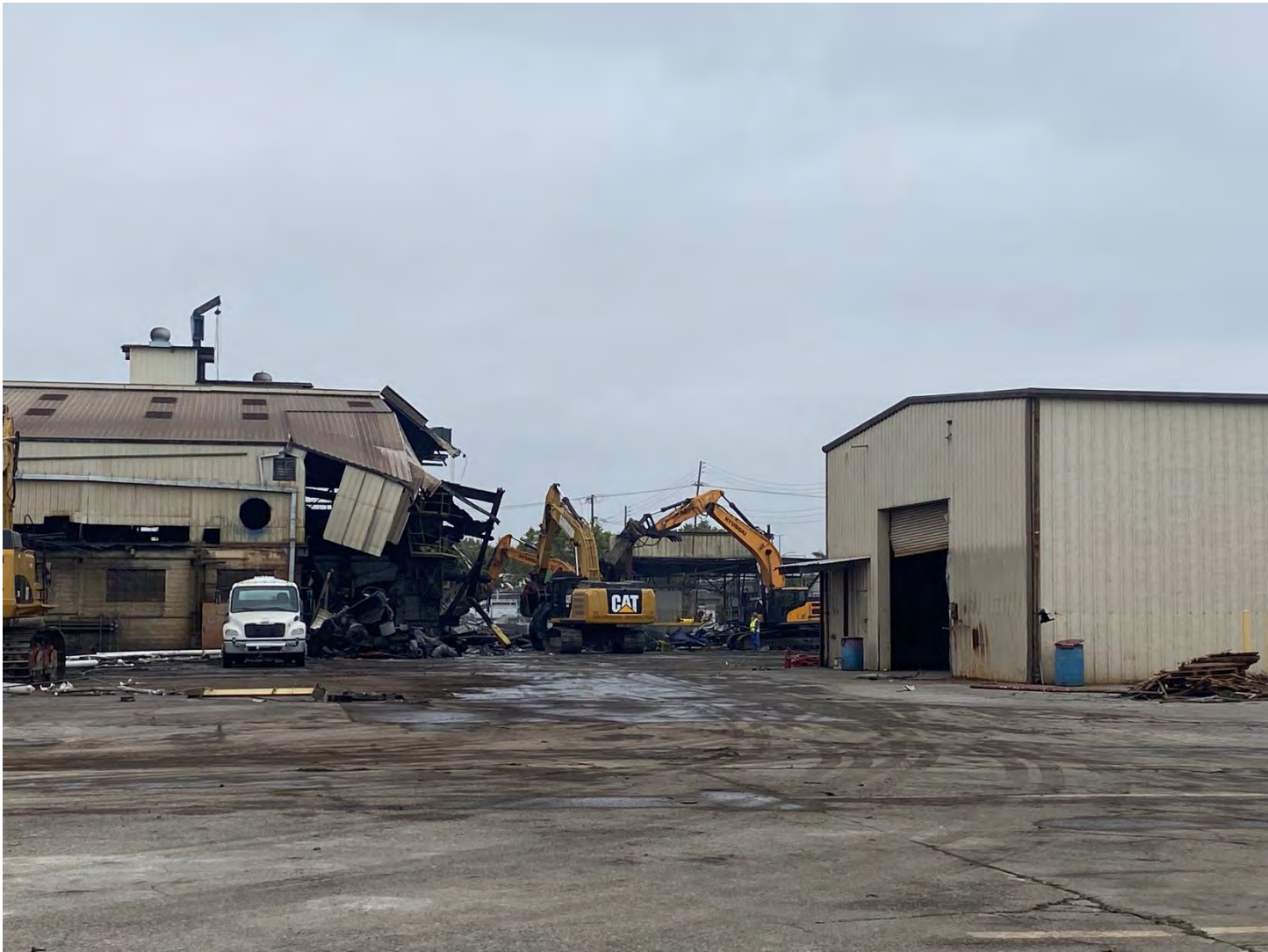
Photo 1: Facing north, demolition of former main facility.
