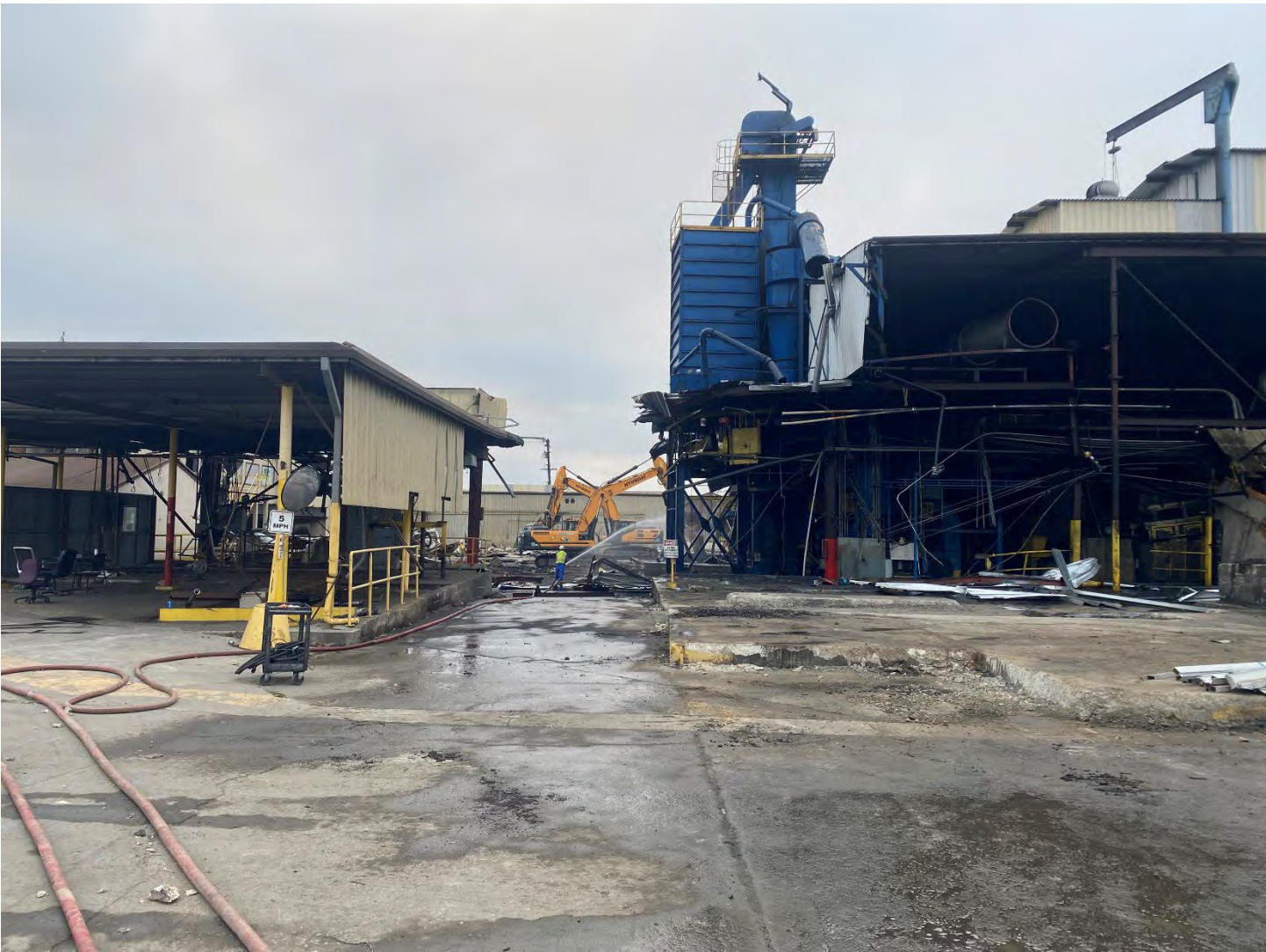
Photo 1: Facing east, demolition of the central portion of the former main building.
