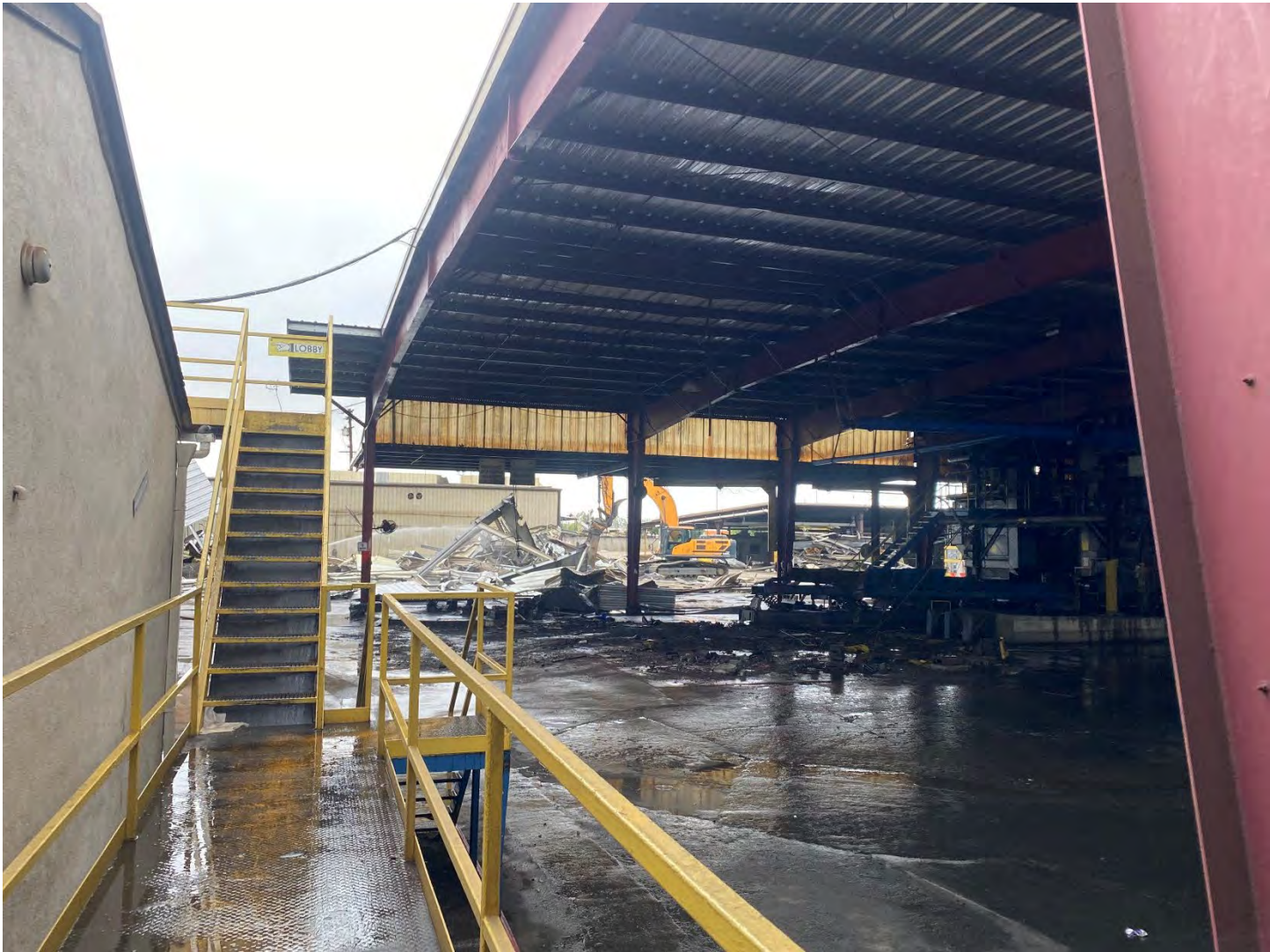
Photo 2: Facing southeast, demolition of the central portion of the main building.
