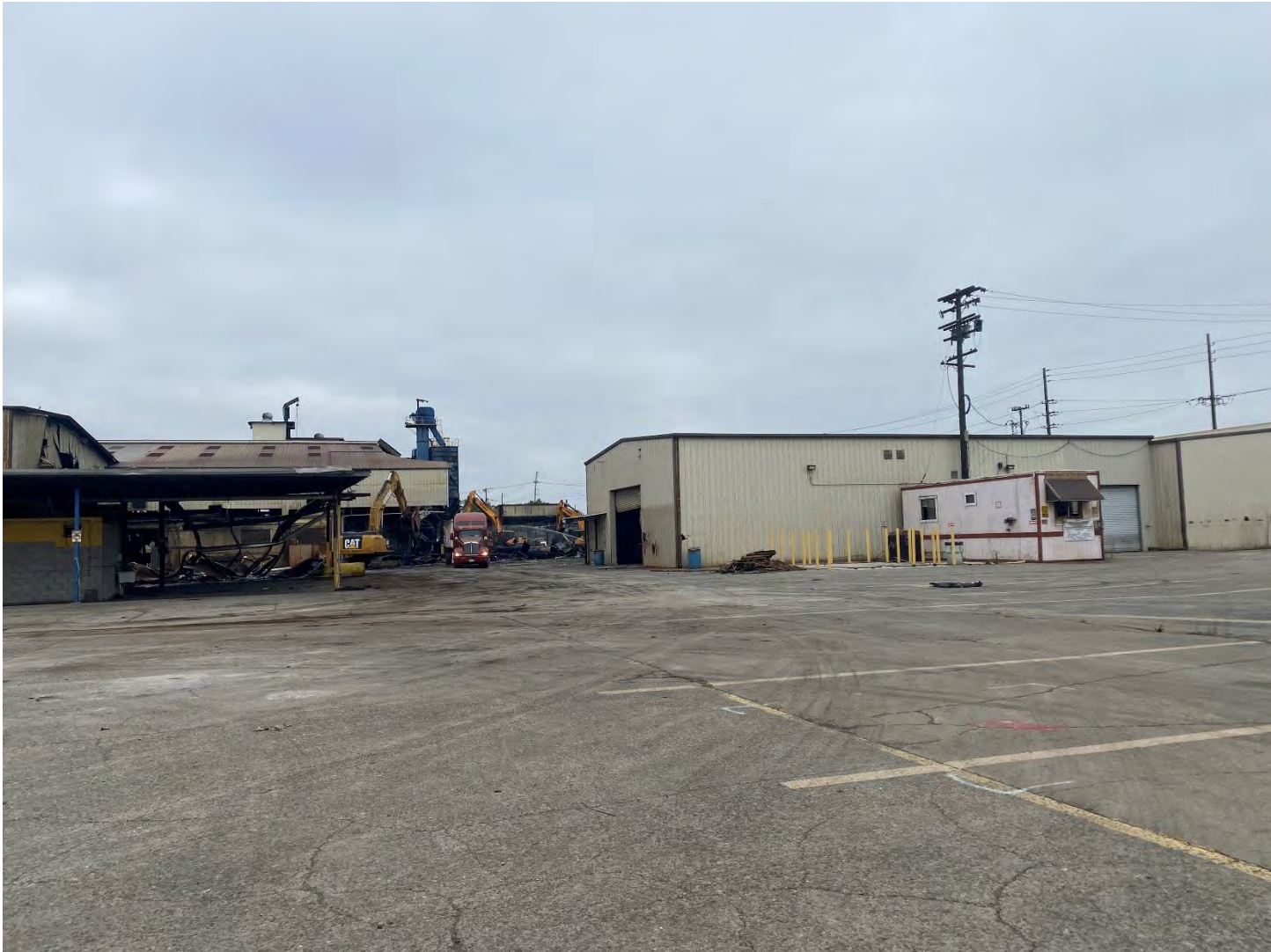
Photo 2: Facing north, loading trucks with demolition debris from central portion of main building.
