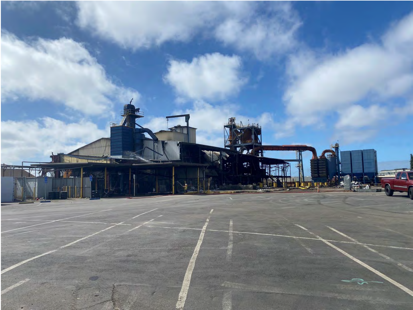
Photo 3: Facing south, water sprayed on portions of main building prior to demolition.
