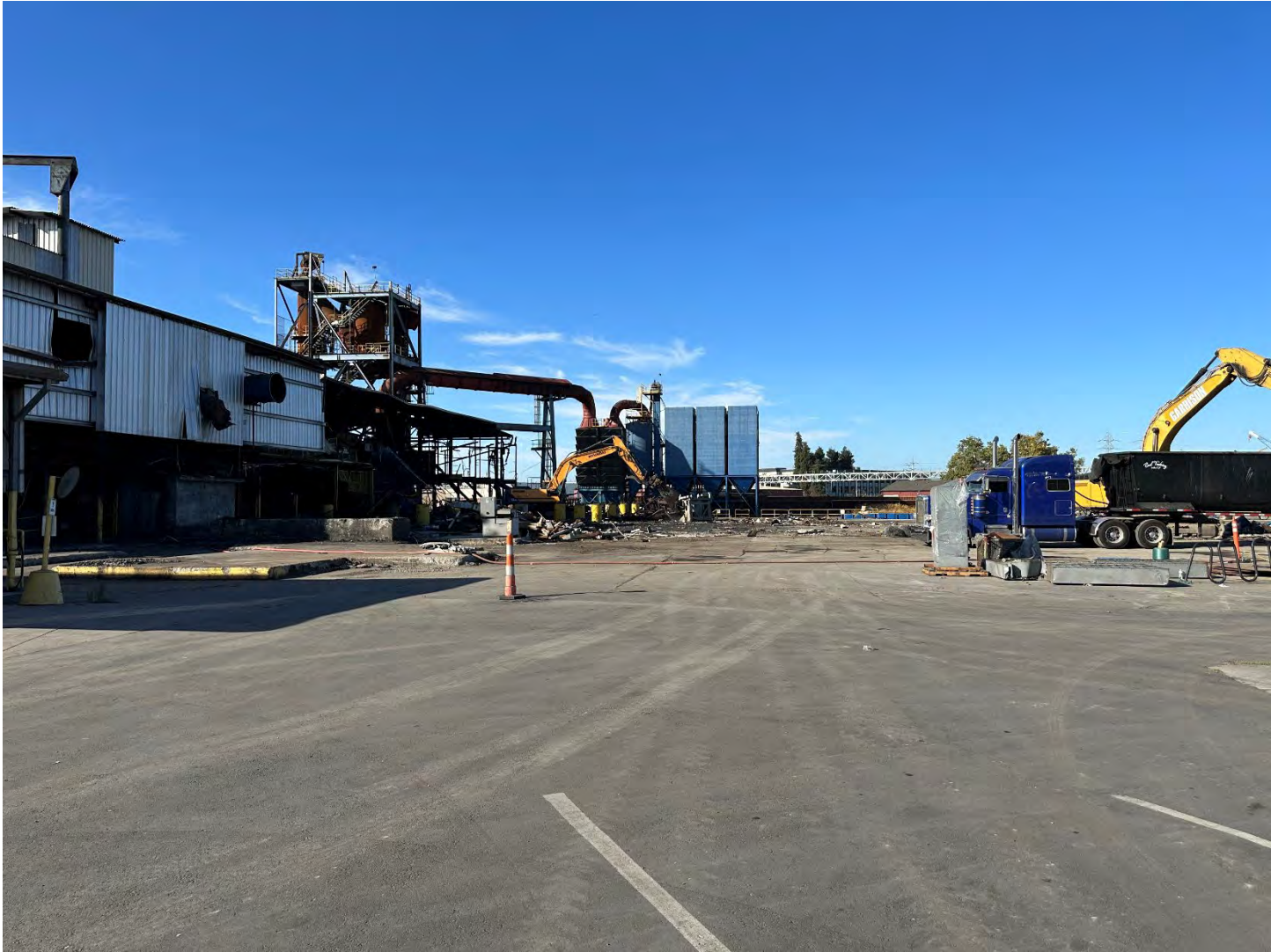
Photo 1: Facing southwest, loading trucks with debris from the Main Facility Demo.
