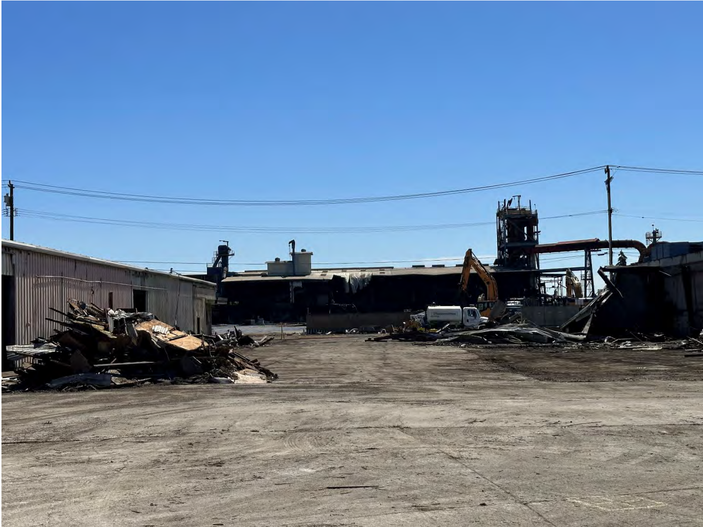
Photo 3: Facing south, demolition progress in the vicinity of the special finishings area with the Main Facility in the background.
