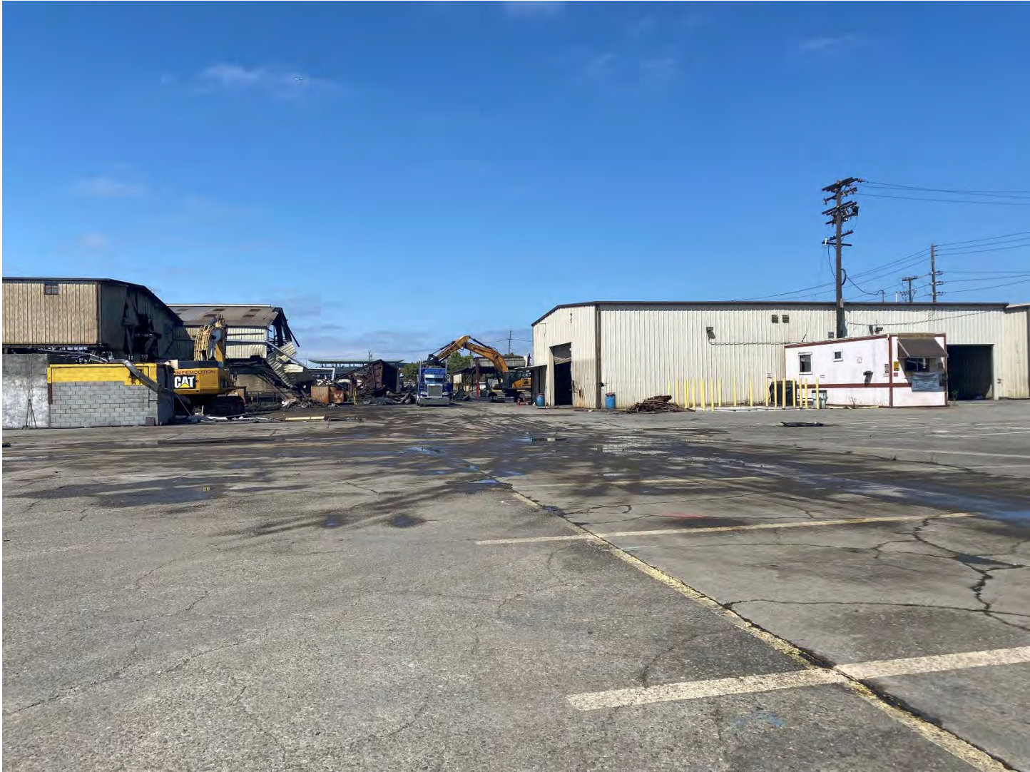
Photo 3: Facing southeast, loading trucks with demolition debris from the former main facility.
