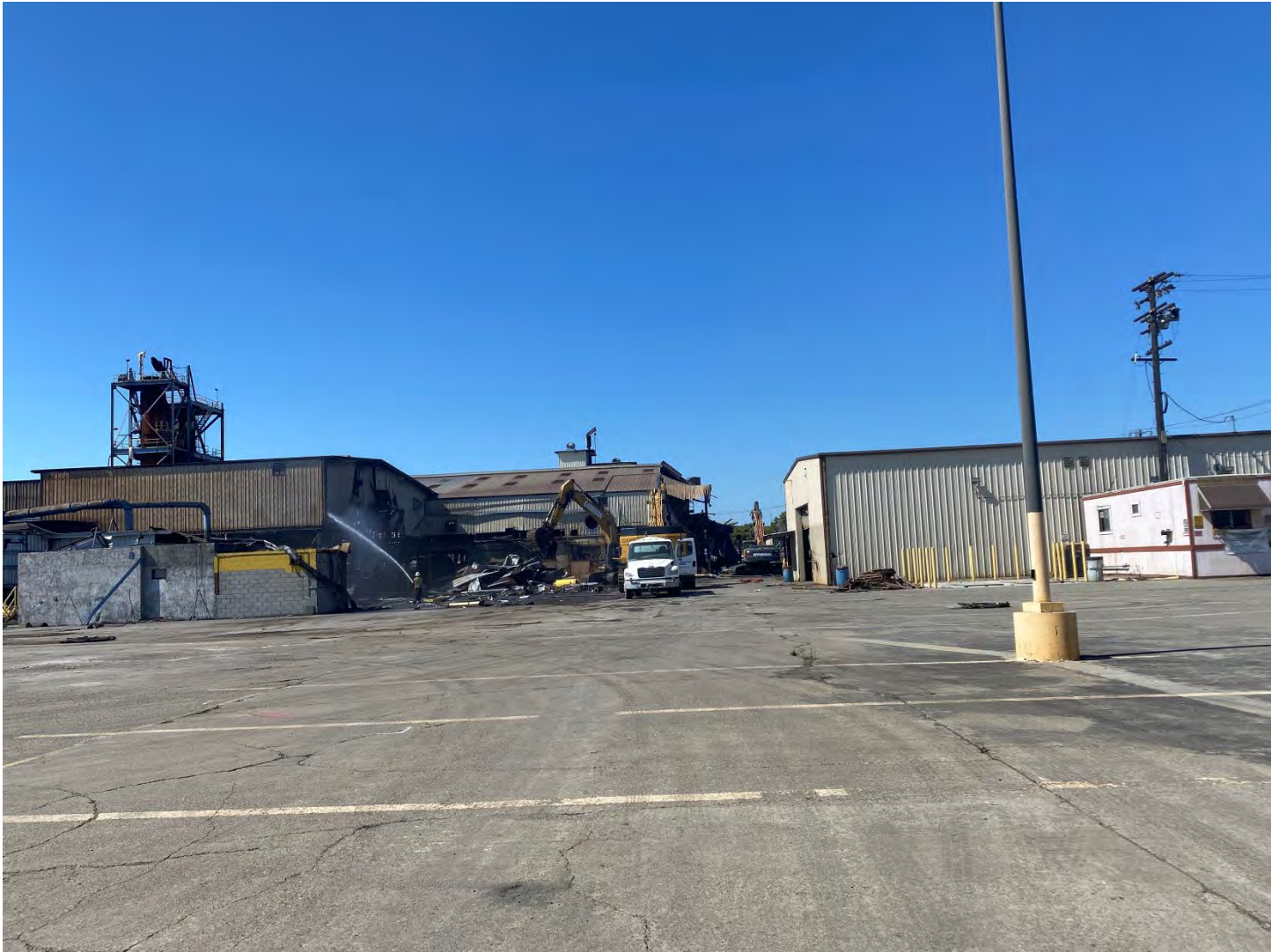
Photo 3: Facing northwest, demolition progress on east side of main building.
