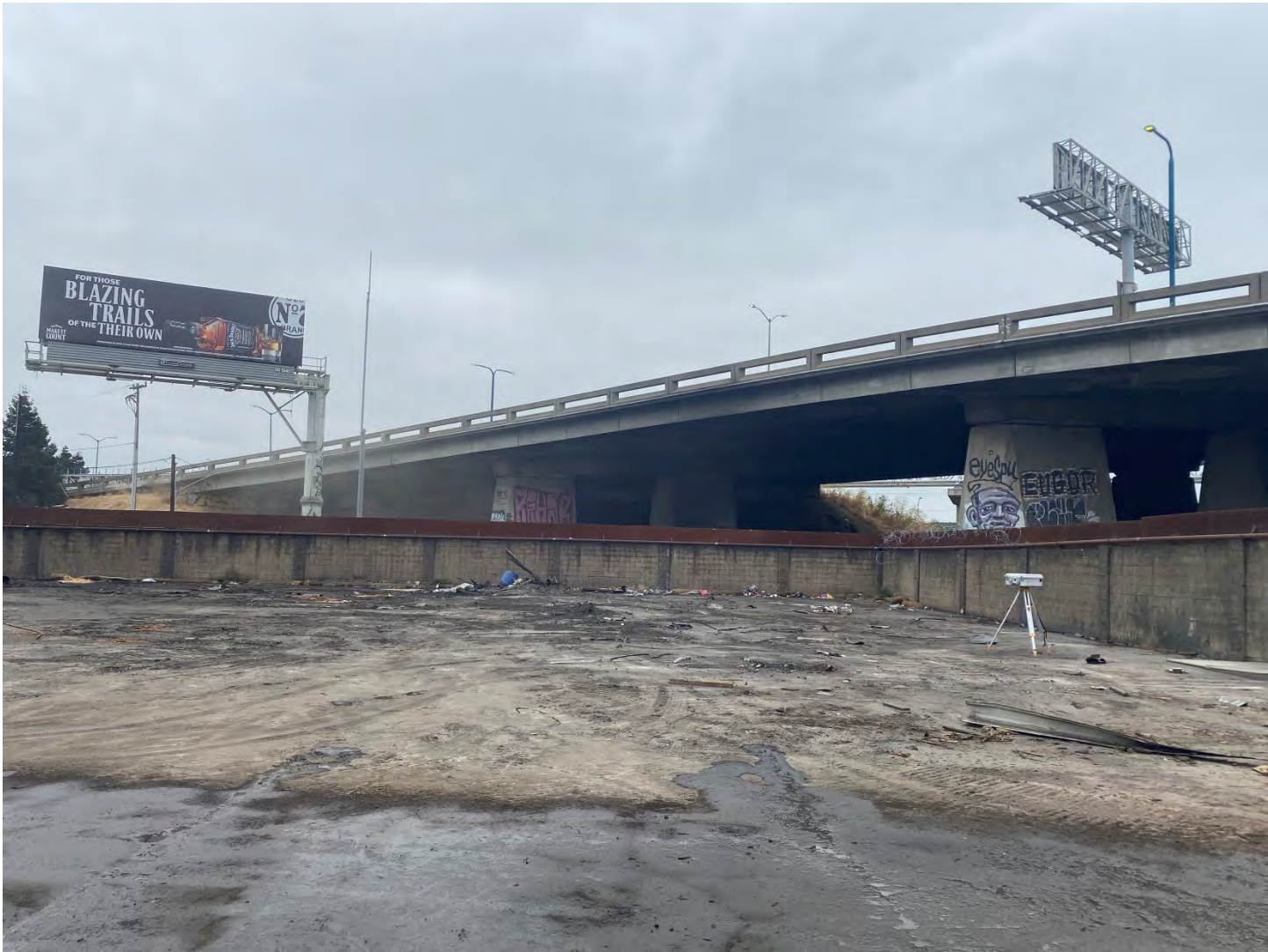
Photo 2: Facing west, visible dust from on offsite source in the vicinity of AMS-02.
