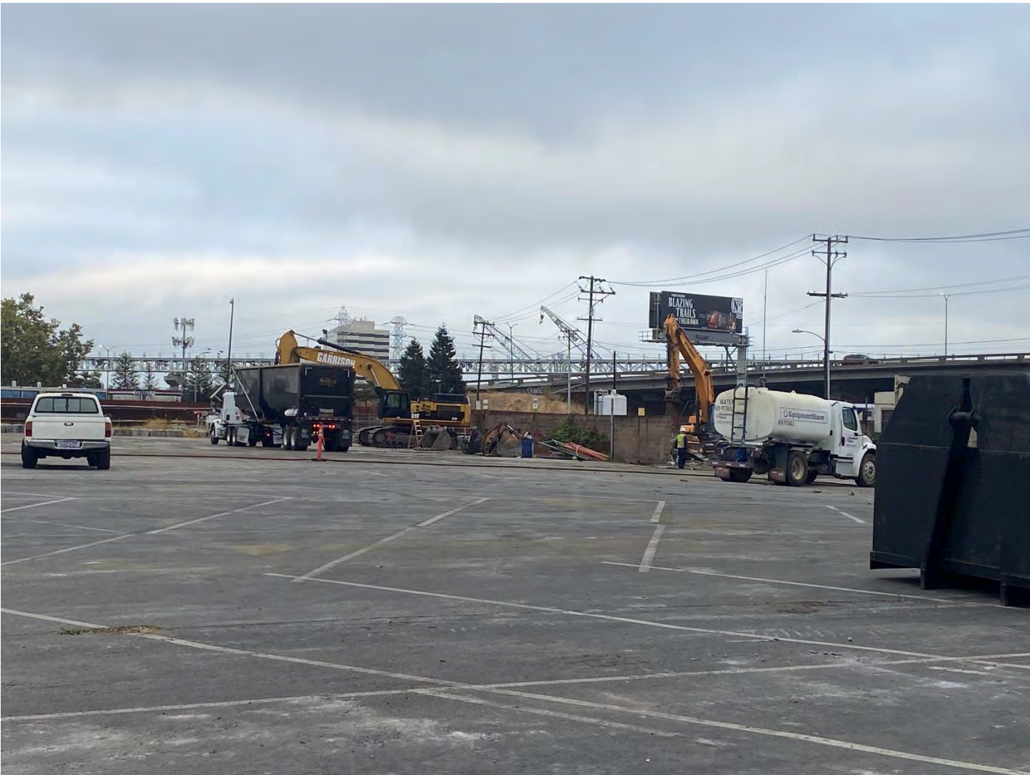
Photo 1: Facing southwest, loading trucks with demolition debris from the special finishings area.
