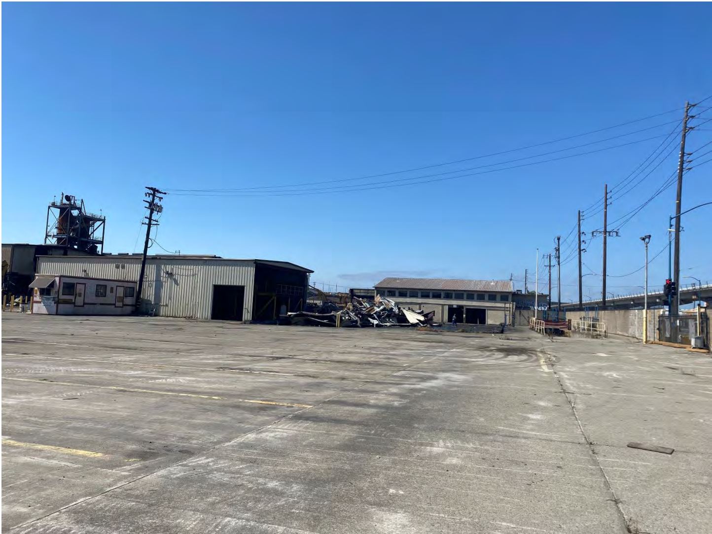
Photo 4: Facing north, demolition progress in the vicinity of the former coreroom and shipping storage area.
