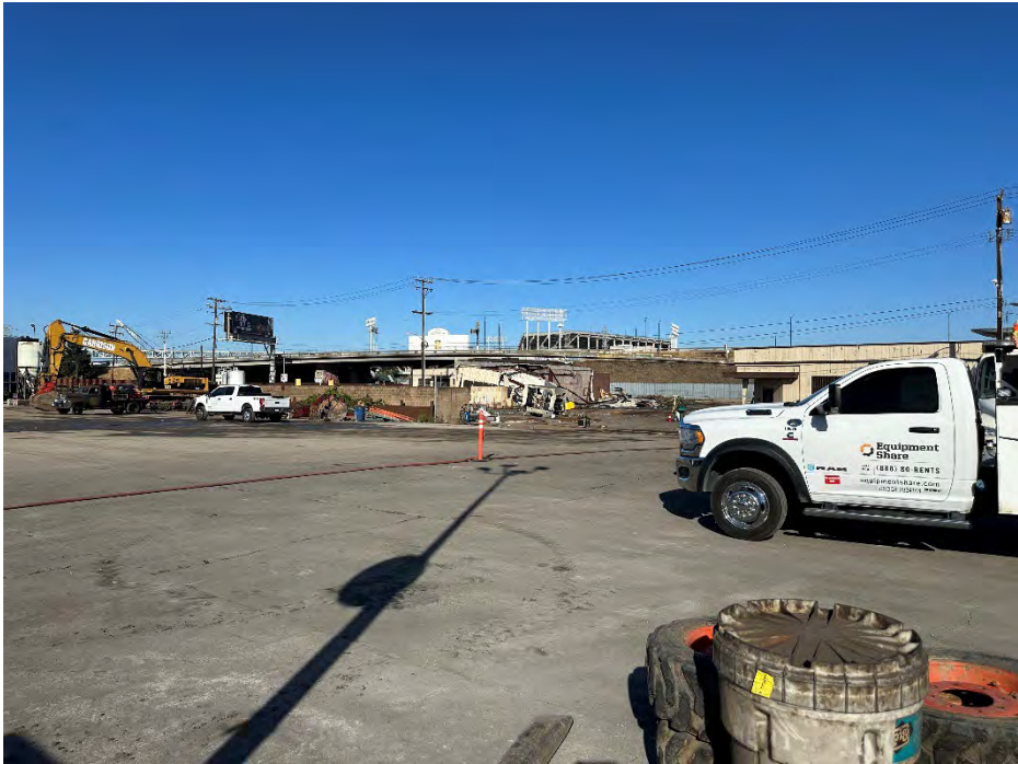
Photo 2: Facing northwest, demolition progress of the Special Finishings facilities.
