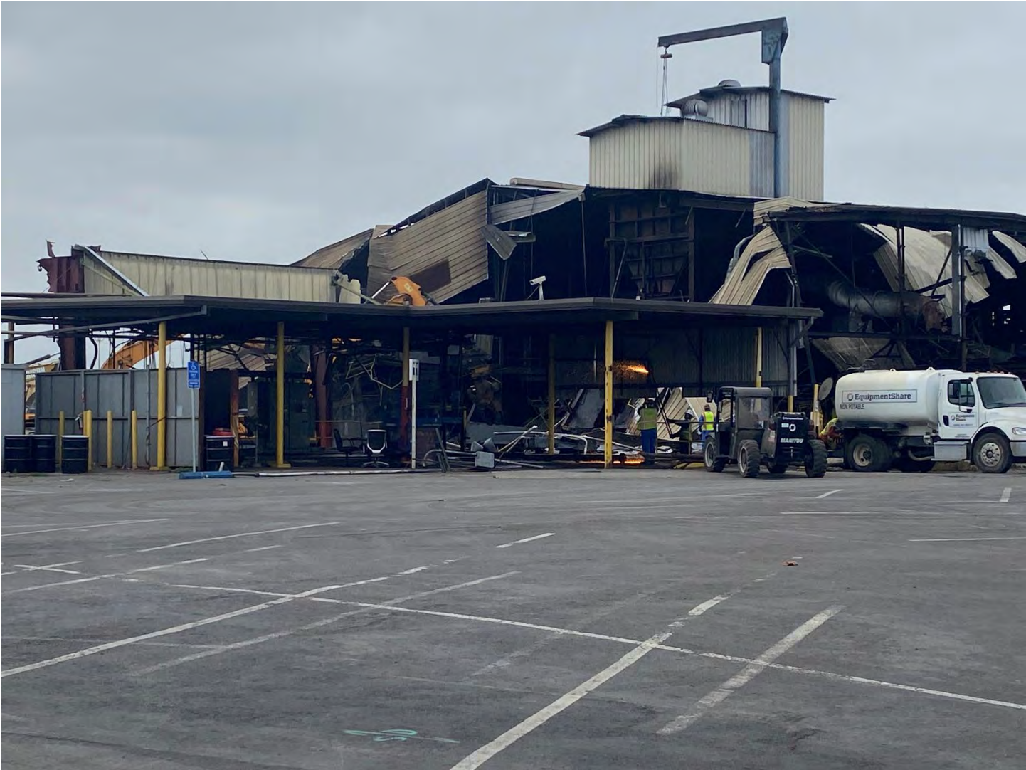
Photo 2: Facing southeast, Hot work activities on the north side of the main facility.
