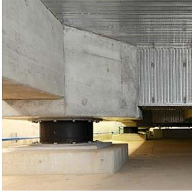
The advanced seismic isolation system is designed to minimize the potential for damage from an earthquake.
