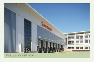
harvested from the roof and generates electricity for use on the site. Air tightness levels exceed U.K. regulations by 75%, while a solar wall and wall-mounted photovoltaic panels generate renewable electricity and provide passive warehouse heating. Carbon credits were purchased to offset the embodied carbon by 110%, creating a net reduction in emissions equivalent to that of more than 440 homes.
