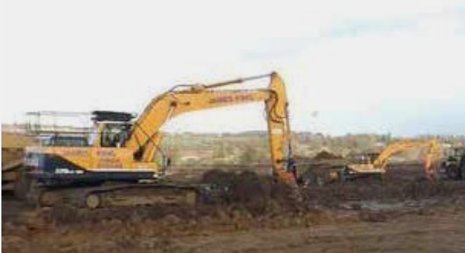
Excavation of the site
