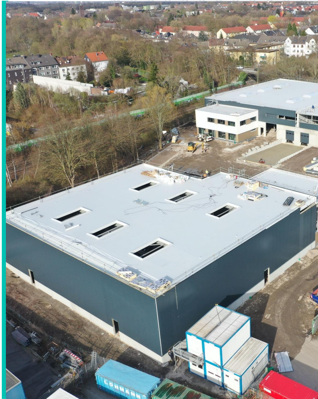
Construction site picture of March 2026
